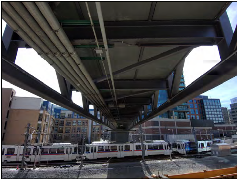
Typical Underside Looking East
