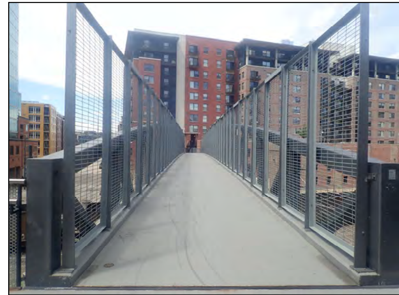
Pedestrian Path Carried Looking West
