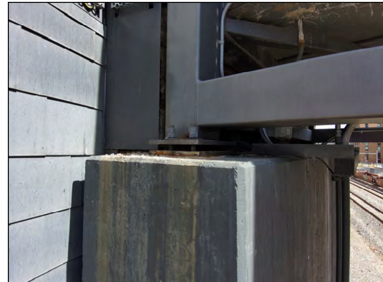
South Moveable Bearing in Expansion at West Pier Looking Northwest
