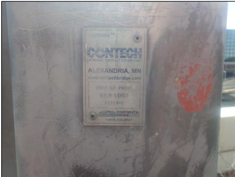
Bridge Plaque at West End of South Truss Looking East
