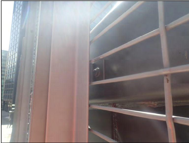
Typical Bolted Connection of Pedestrian Rail to Truss Looking East
