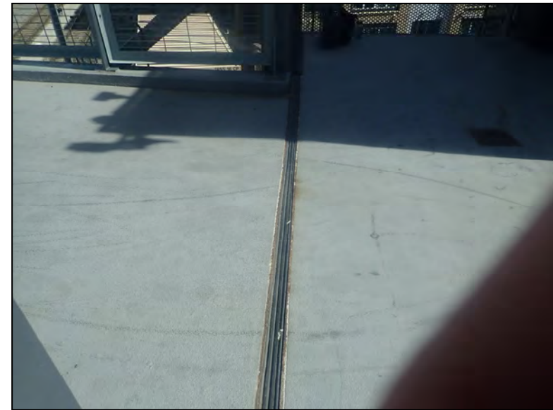
East Compression Joint Looking North
