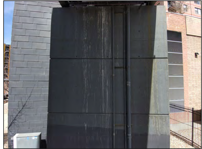
West Pier Looking West
