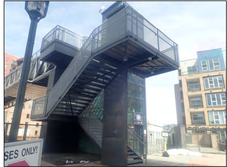
Overall View of East Stairwell Looking Northwest
