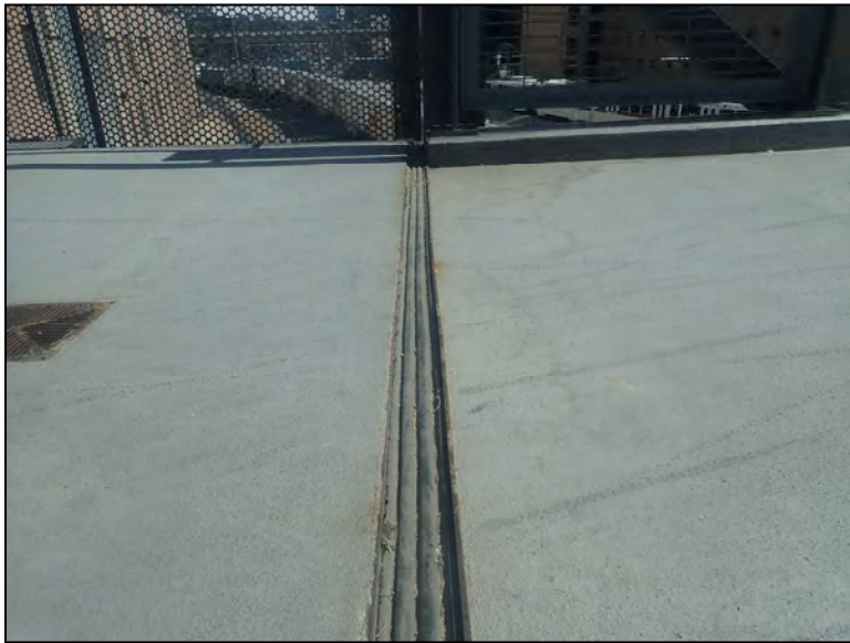
West Compression Joint Looking North
