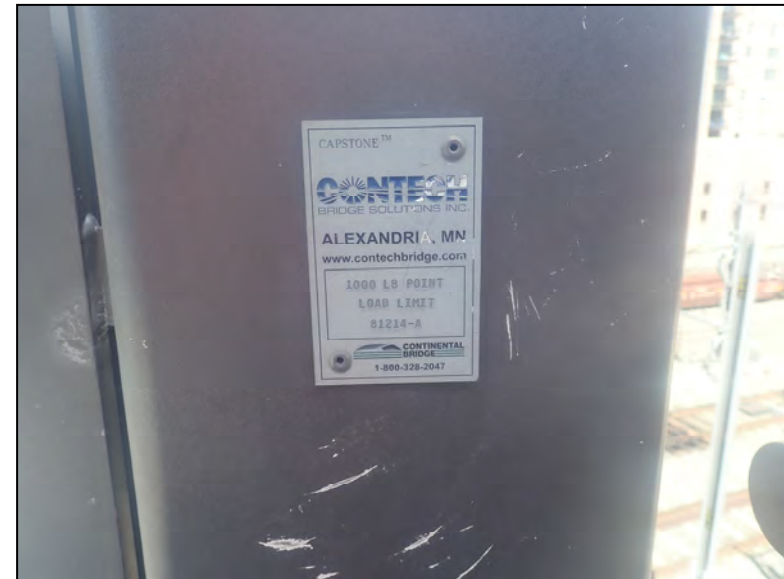
Bridge Plaque at East End of North Truss Looking West
