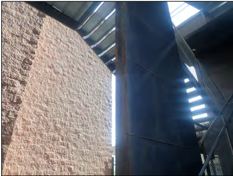
Architectural Panels at Stairwell Columns Looking Northeast
