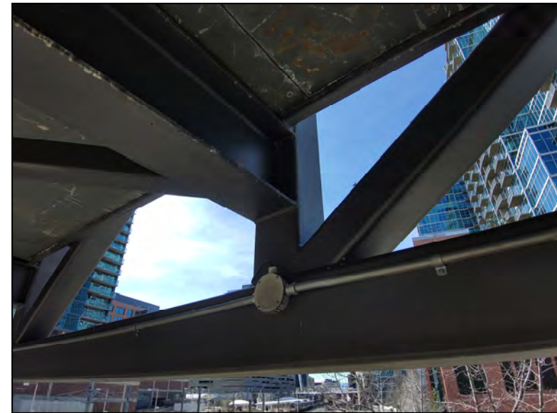
Typical Lower Chord and Floor Beam Looking Southeast
