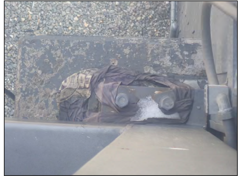
North Fixed Bearing at East Pier Looking North
