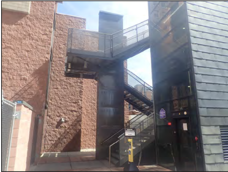
Overall View of West Stairwell Looking North
